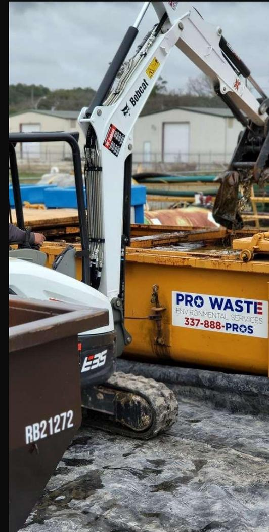
CCCP-7010SC TriBlend was mixed with the oily-water emulsion to reduce disposal costs by about \$10,000 per roll-off box volume.
